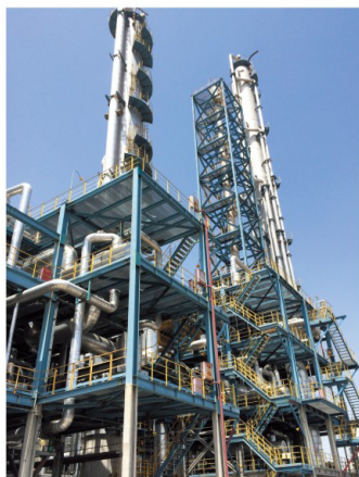
8 Sets of Coil-Wound Heat Exchanger in Rectisol Process System for Coal to Hydrogen Complex
