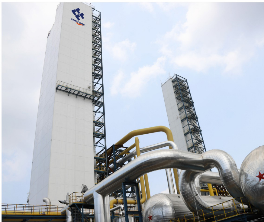
GOX60,000Nm 3 /h (2,000TPD) + GOX30,000Nm 3 /h (1,000TPD) ASUs for Steel Making Complex
